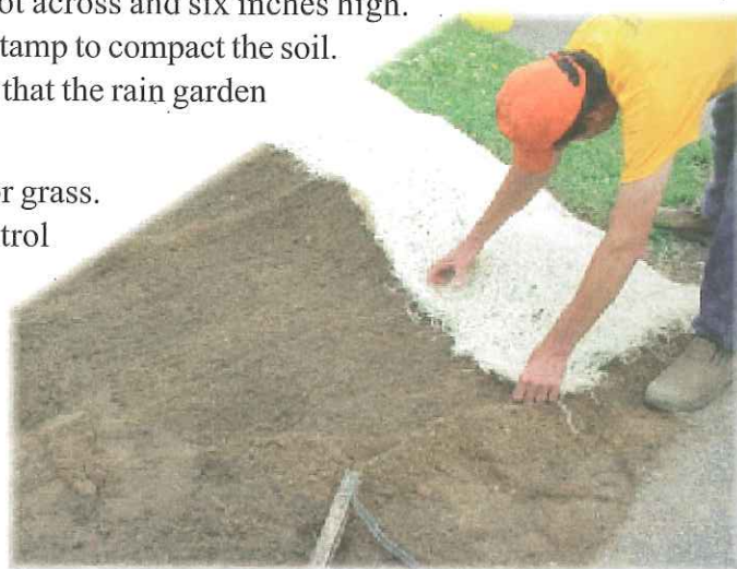
Erosion control matting made of coconut fiber is carefully placed along the berm to prevent erosion on the downhill side of the rain garden.
